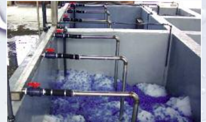
Biological waste water treatment plant for cleaning stations.
