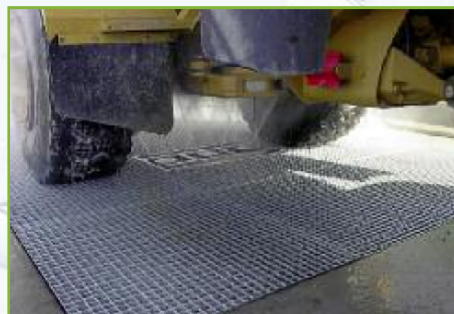
Under chassis cleaning.
