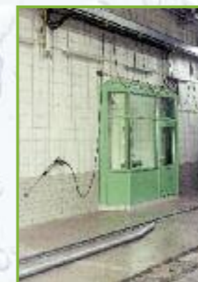
Hose trolley system.
